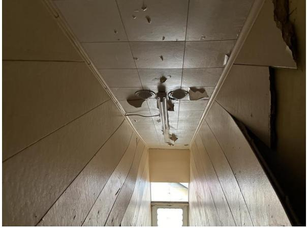
A photograph of a ceiling in a stairwell. The ceiling is made of metal and has several rectangular fluorescent light fixtures. The ceiling is in a state of disrepair, with some holes and missing sections. The walls are made of wood paneling.                                            |
